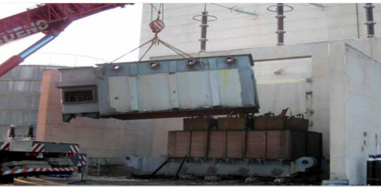
Dismantling of the main transformer
