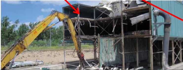
Demolition of the cooling towers
